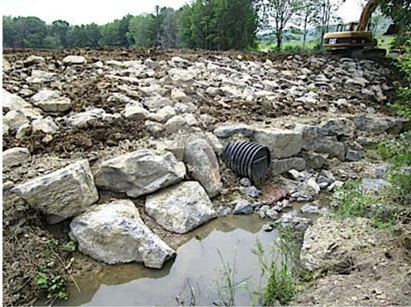
During inspection of the site, it was noticed that the dike itself was in very poor condition. This was due to water breaching the dike many times, as the outlet control structure had not been functioning properly for some time. It was also noticed that the earthen, emergency spillway had eroded severely and the only thing that would retain the water in the wetland (even with a functioning, primary outlet control structure) was an existing beaver dam.
